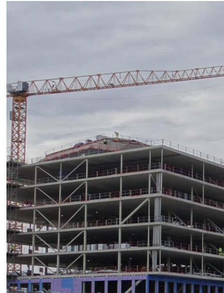
Park Central – Garage
